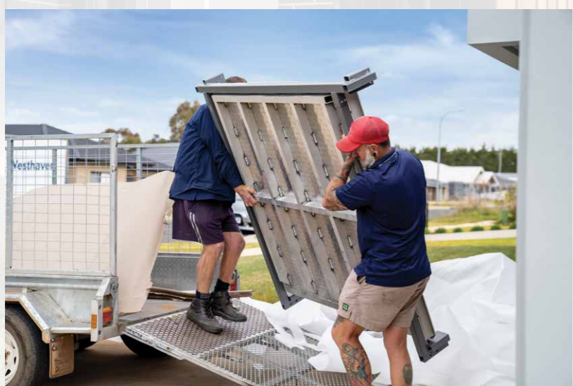
Ramp installation at a Westhaven property.
