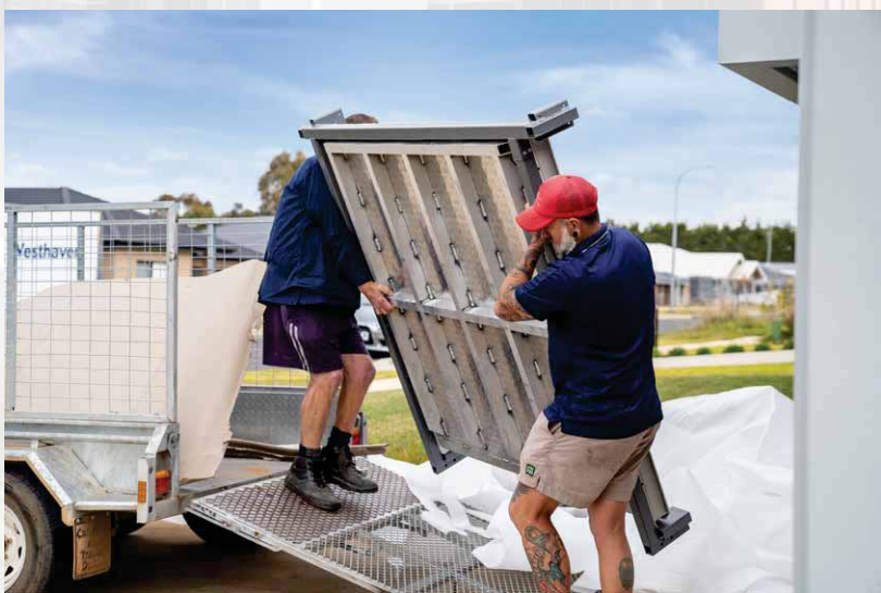
Ramp installation at a Westhaven property.
